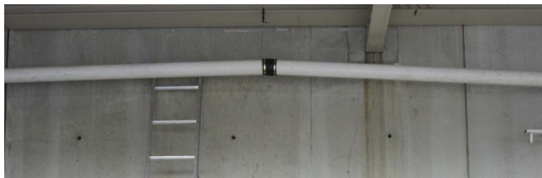
DO NOT pitch pipes upward.
