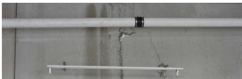
Keep pipes pitched downward.
